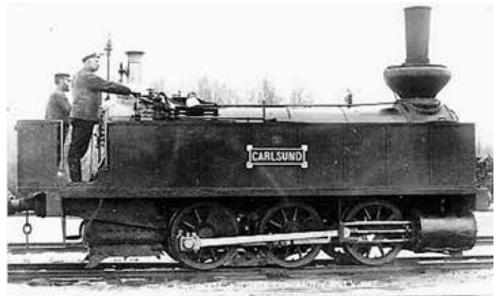
The company's first locomotive. The train transported ore from Zinkgruvan to Åmmeberg. It brought back coal to Zinkgruvan's steam-powered machines.
